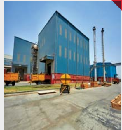
Biomass Based Steam System, Rohad
