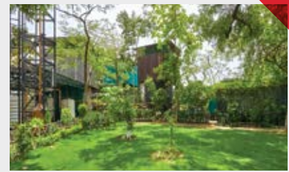
Bio compost and Biogas unit, Hapur
